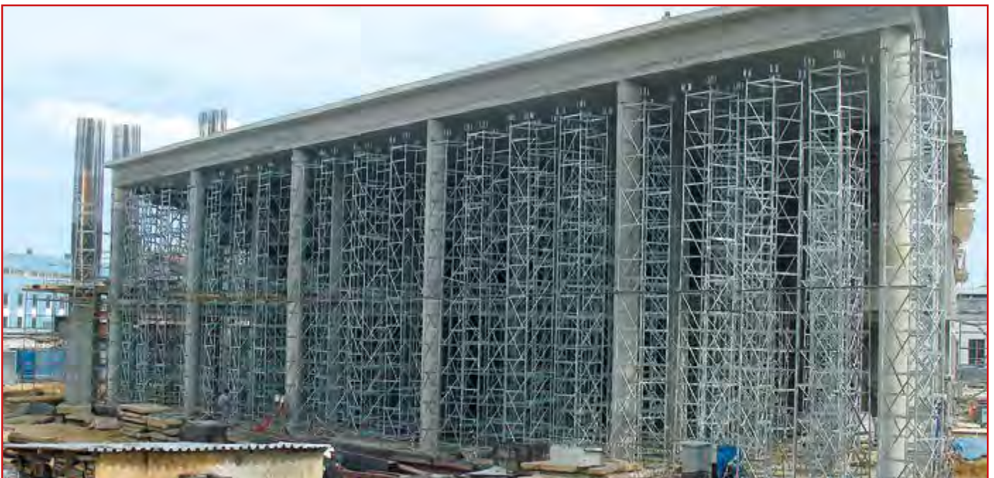
S10 supporting tower – diagram
