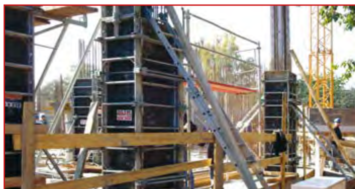
Pole forming – MIDI BOX boards and formwork locks
